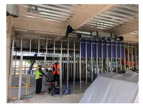
Photo 5 – Building A Corridor with MEP components, wall framing, and some sheathing installed.
